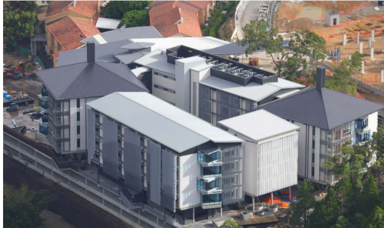
Dovetree aerial view (also showing the early construction of Rosemount Retirement Living)
